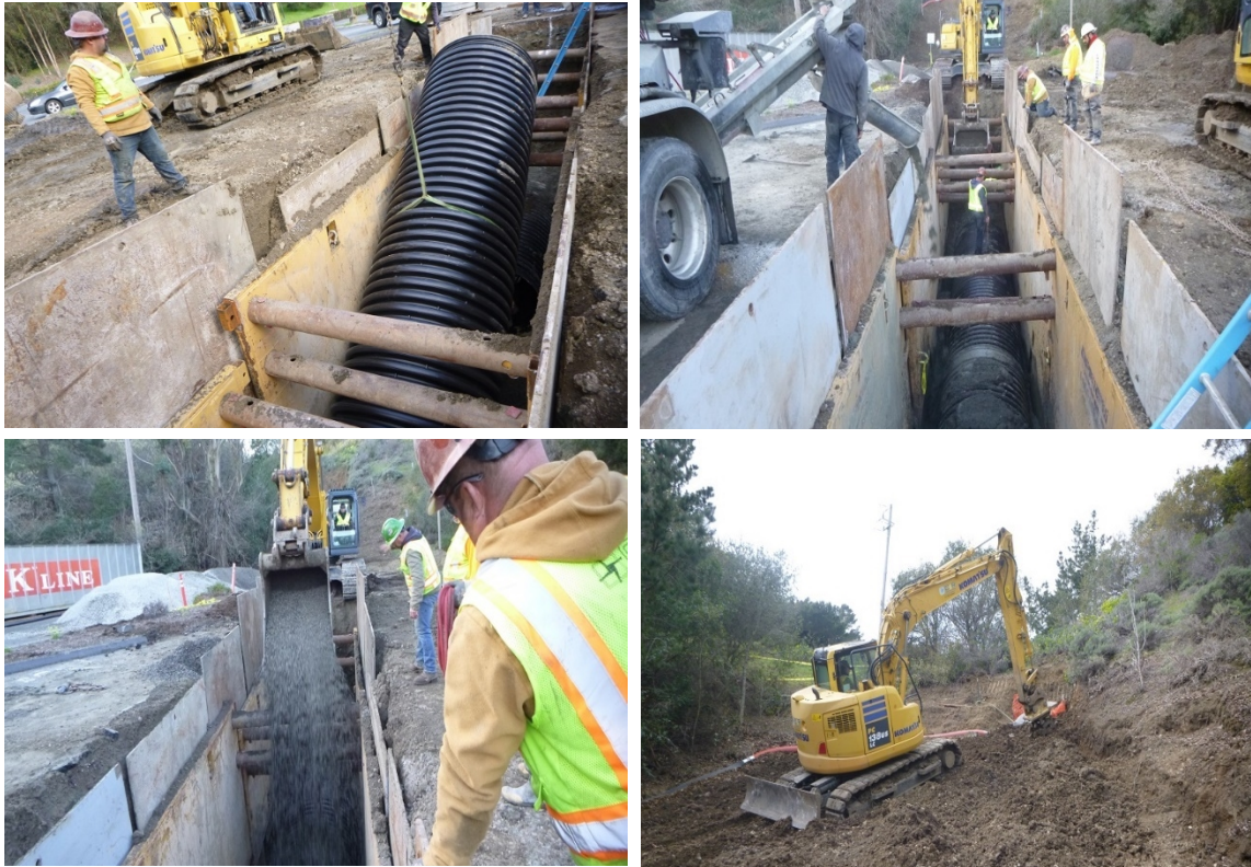
Figure 1 – Completion of Pipe Replacement at the Northwest Corner of Skyline Boulevard and Sneath Lane
